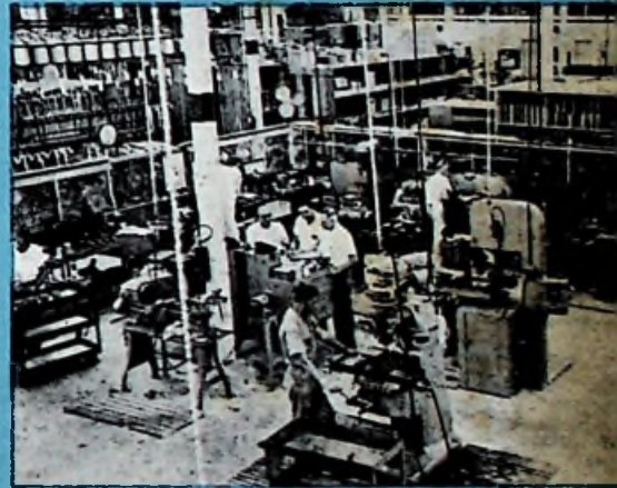
The equipment in the Tool and Die Department in Perko's new Miami plant is overshadowed by the caliber of men who man it.
